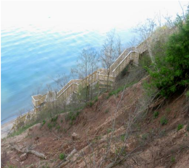
Circuitous New Stairs at Virmond Park's Lake Michigan Beach in Mequon, WI. The Bottom Section Lifts Up to Avoid Winter Waves and Ice.
