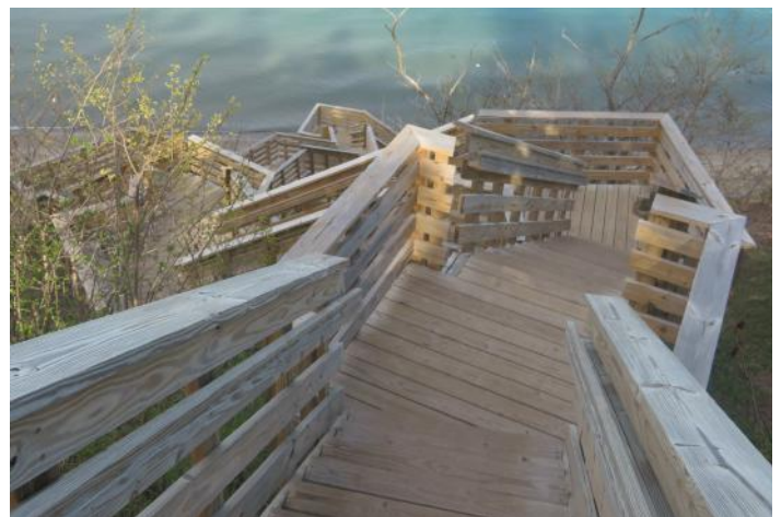
Circuitous New Stairs at Virmond Park's Lake Michigan Beach in Mequon, WI. The Bottom Section Lifts Up to Avoid Winter Waves and Ice.
